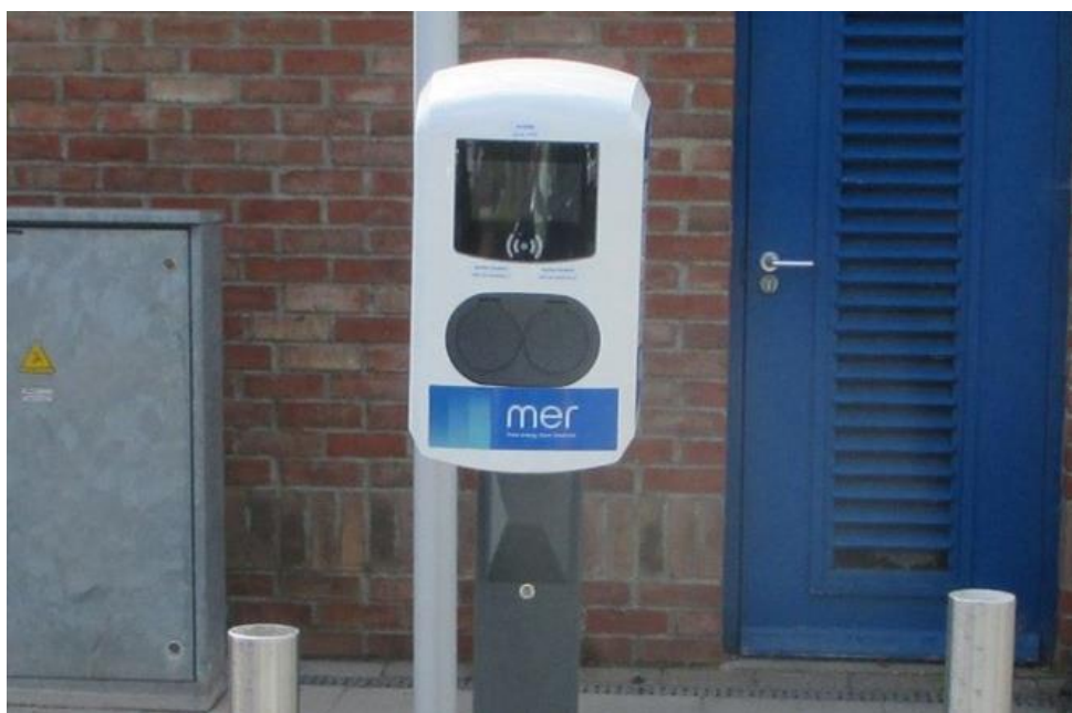
Figure 17: Task 3 Chargepoint with 1065mm socket-height with visible screen reflections
