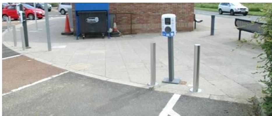
Figure 14: Task 2 location with 940mm height socket device and bollards arrangement
