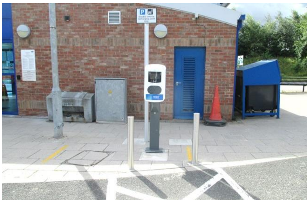
Figure 15: Task 3 location with 1065mm height socket device and bollards arrangement.
